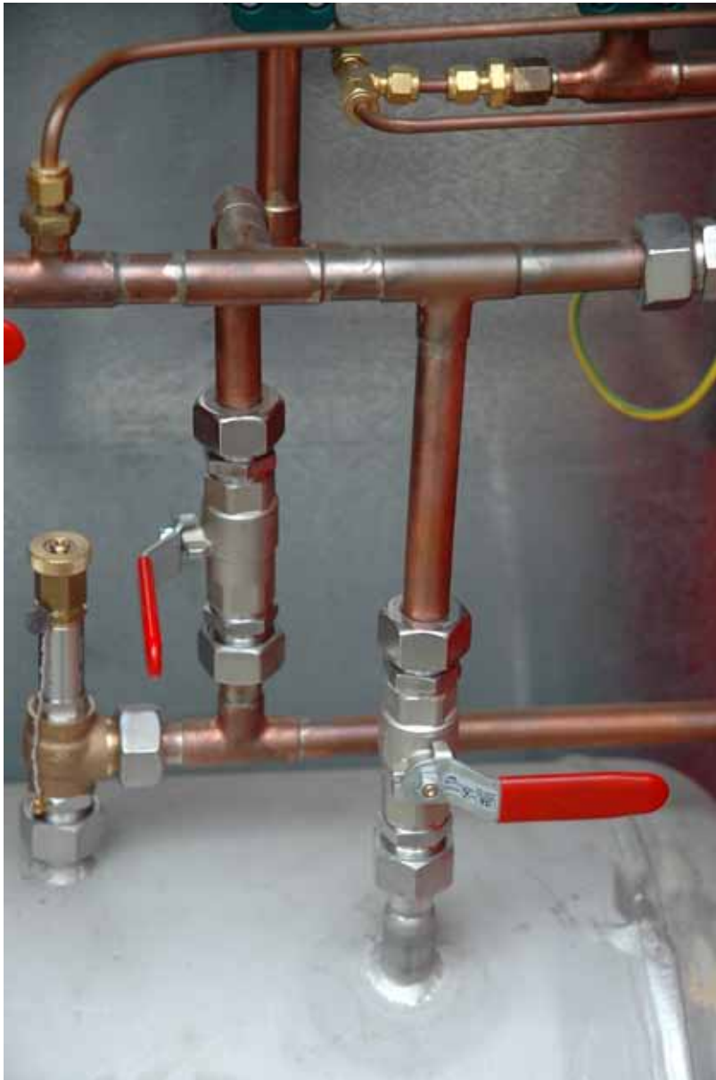
Fig.: Gas pipes made of copper
