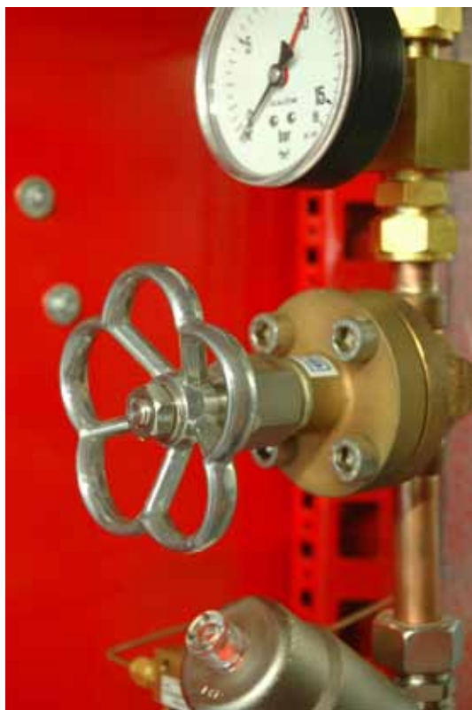
Fig.: Stuffing valve
