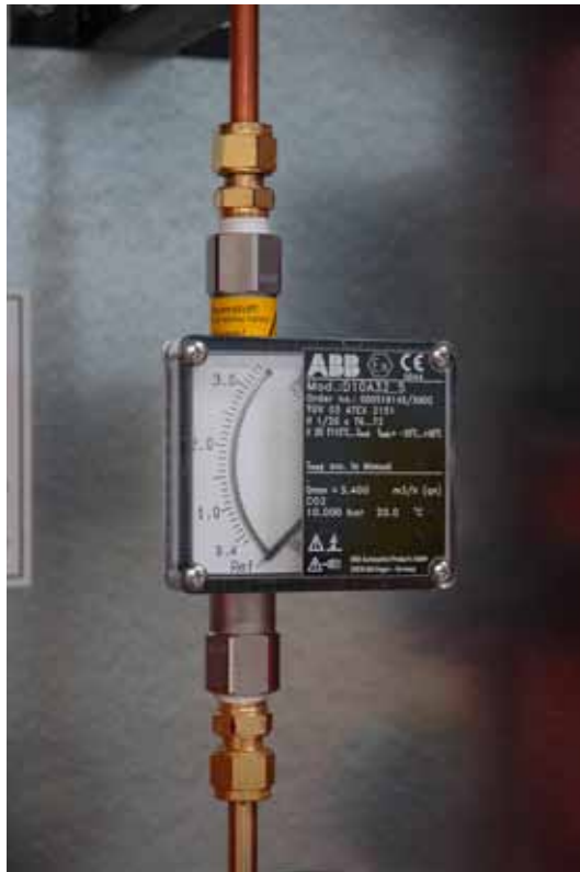
Fig.: Flowmeter for additive gas
