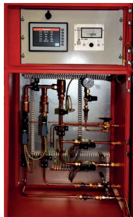
Figure 2. Lean air system with SIL 1 gas analyser
